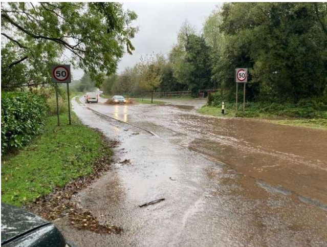
Figure 3: September 24, Flooding at Linby Lane
